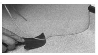
Allow the weldrod to cool completely, then trim surplus with the spatula. Chamfer off the external mitre with the square router blade.
