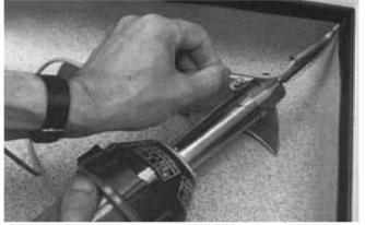
1. Groove the lower section of the joint, but not the upper.
